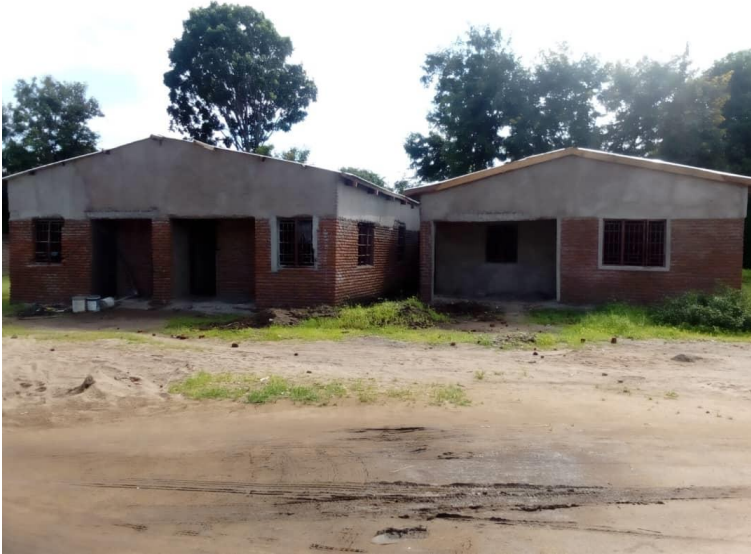
Teachers house on the right, under construction at Everland
