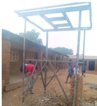
Construction of the water tower.
