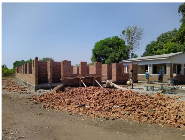
Construction of the maternity wing Underway
